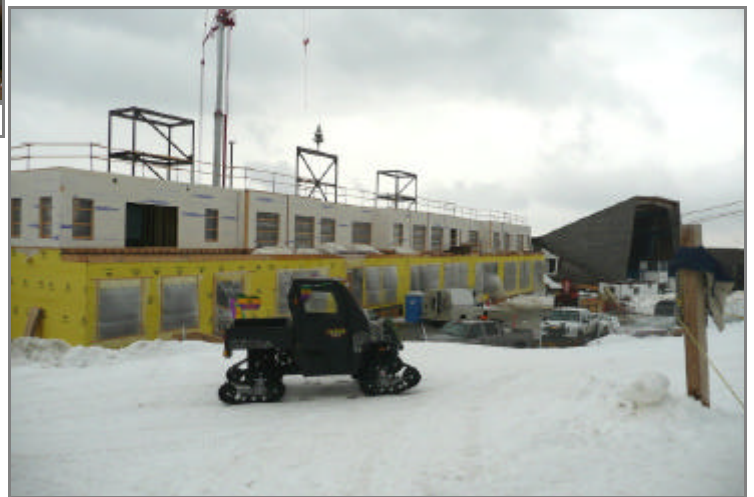
The new Hotel Jay under construction—finally!
